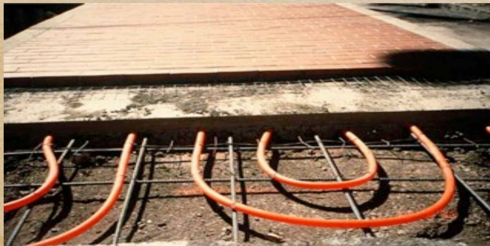
Geothermal radiant heating
